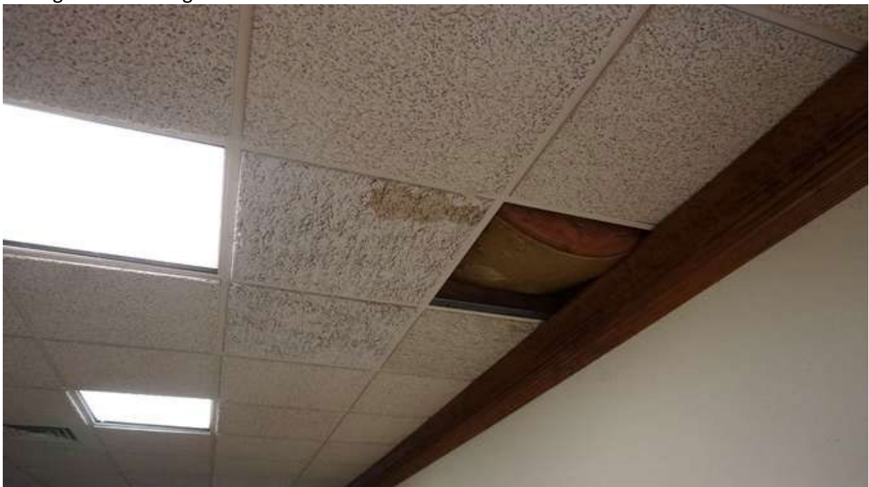
Ceiling Water Damage
