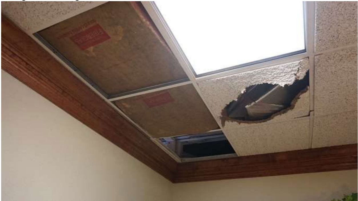
Ceiling Water Damage
