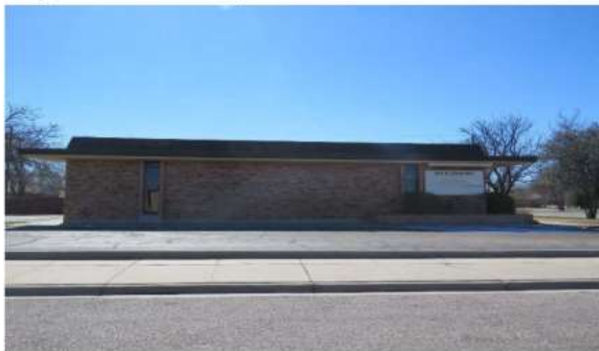
Photograph 4: North elevation of the subject roof.
