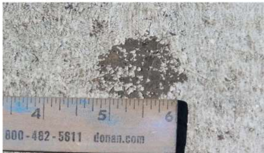
Photograph 34: The paint-covered, modified bitumen membrane circular paint-chips without fractures.
