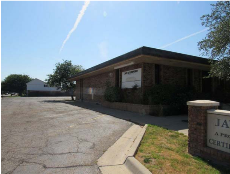
LEFT VIEW FACING SOUTHEAST
