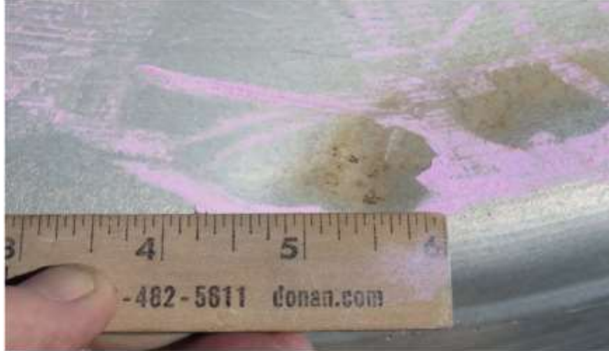
Photograph 17: Close-up of the dents on the powered blower.
