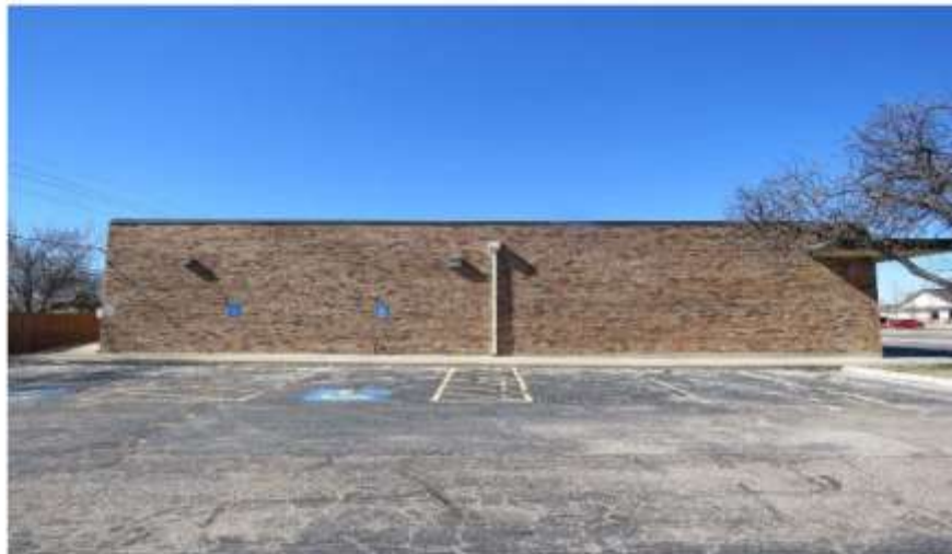
Photograph 3: East elevation of the subject roof.
