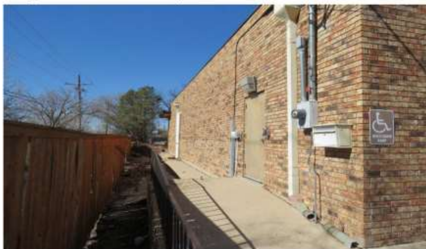
Photograph 2: South elevation of the subject roof.
