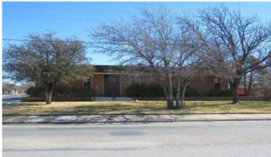
Photograph 1: West elevation of the subject roof.
