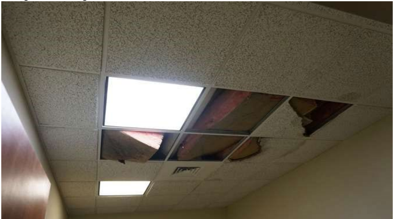
Ceiling Water Damage
