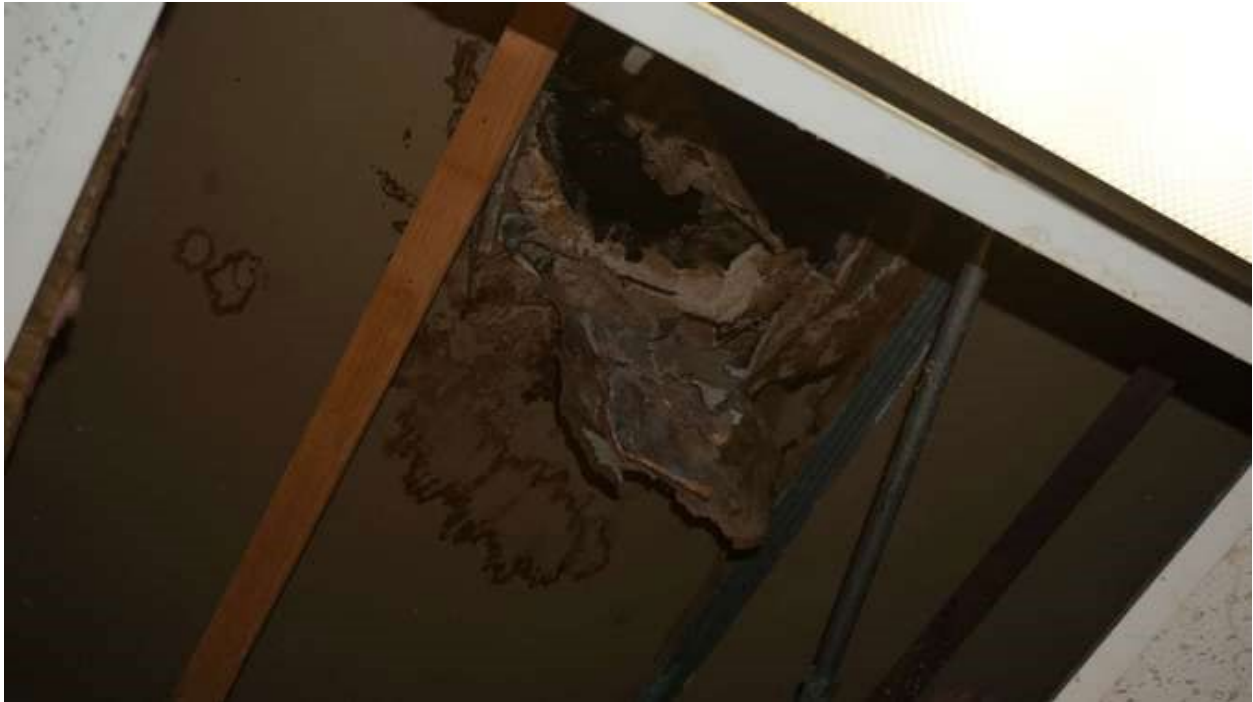
Roof Leak
